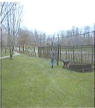
Installing new ornamental fencing at Shellabarger Park.
