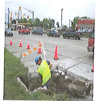
Rebuilding catch basin on Linden Ave.
