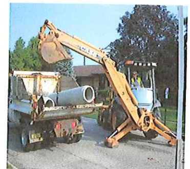
Replacing damaged storm sewer pipe.
